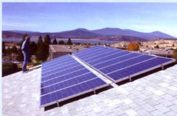
A rooftop 2.5 KW photovoltaic grid-tied array provides solar power for the University Advancement building (formerly the daycare center) at Oregon Tech.
