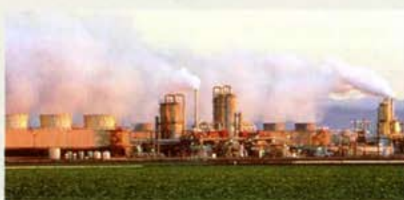
Geothermal energy is generated by tapping into hot steam that lies beneath the earth's surface. There are 69 geothermal power plants at 18 different sites now operating in the U.S. Geothermal plants emit little air pollution and provide more than 2,700 megawatts of power — the equivalent of three large coal-fired or nuclear power plants and enough to provide electricity to 3.5 million homes. "Each year the United States saves 22 million tons of carbon dioxide, six million tons of carbon, 41.5 million barrels of oil and 200,000 tons of sulfur dioxide," says John Lund, director of Oregon Tech's Geo-Heat Center. Geothermal resources come in five forms: hydrothermal fluids, hot dry rock, geopressured brines, magma and ambient ground heat. Of these five, only hydrothermal fluids have been developed commercially for power generation. The state and temperature of water in a reservoir determines what type of power plant can be built. To learn more about geothermal power, visit the Geothermal Resource Council ( www.geothermal.org ), Geo-Heat Center ( geoheat.oit.edu ), Geothermal Education Center ( geothermal.marin.org ) or U.S. Department of Energy ( www.eere.doe.gov/geothermal ).
